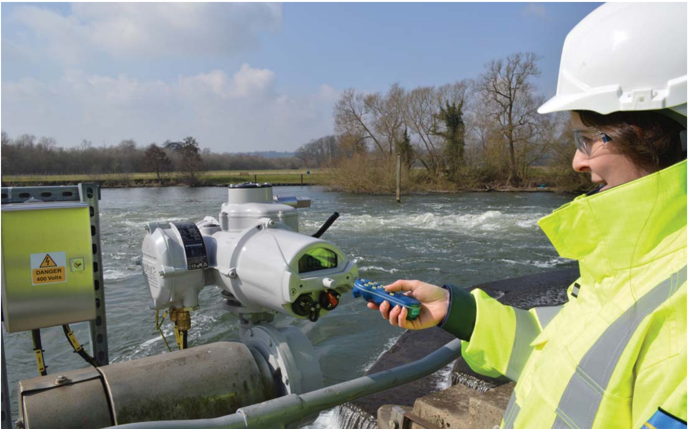
Fig 2 - Using the setting tool, information stored in the dataloggers of up to ten IQ actuators can be downloaded and transferred to a PC for analysis and diagnostic purposes.
